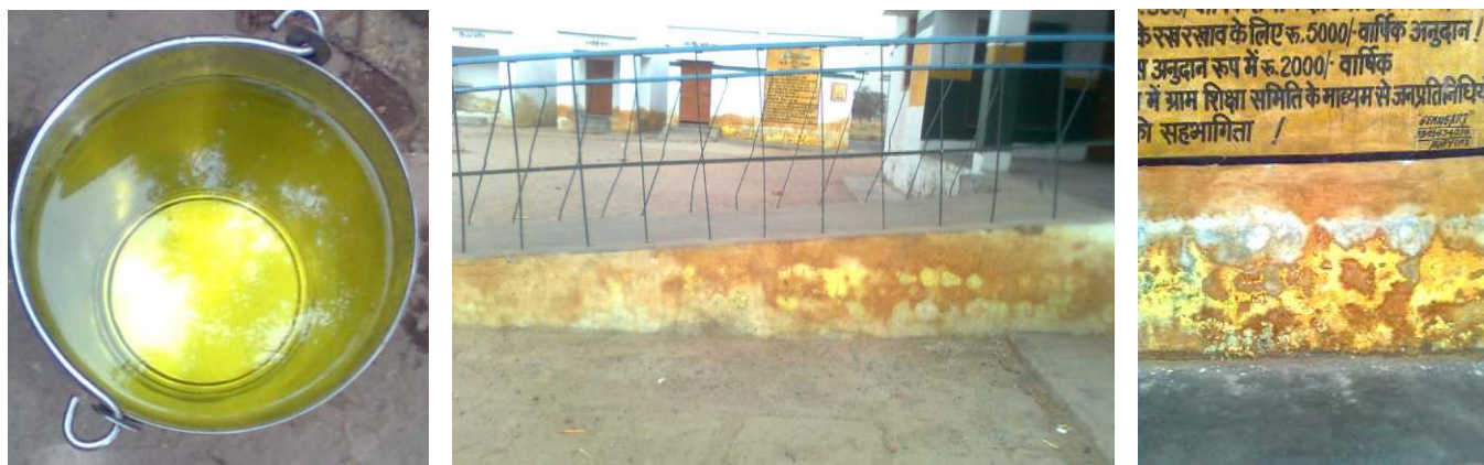
Fig: Left : Groundwater with pale yellow color imparted by high Cr (VI), Middle, Right : Impact of chromium leaching on the walls of building constructed in area where chromium rich sludge was dumped used for land filling.
